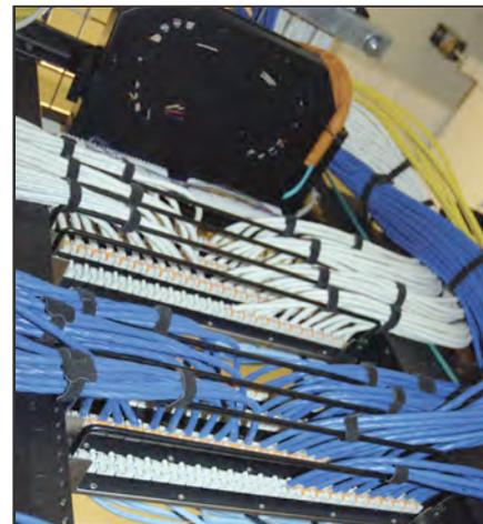
Belden's FiberExpress fiber backbone (Orange cable) runs from the Computer Room to each floor's telecommunications room. The 10GX copper-based cables (Blue, White and Yellow) run horizontally to deliver high-bandwidth 10 Gigabit to desktops on all floors. All fiber links have redundant pathways built in to ensure maximum reliability and network uptime.
